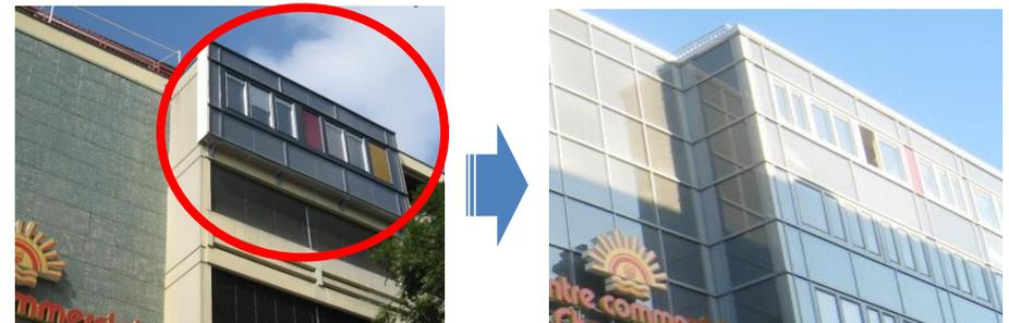
Pre-fabricated solar facade system from gap-solution
