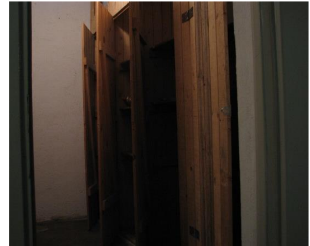
Before renovation – basement storerooms
