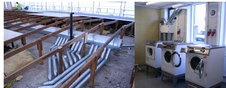
Installation of ventilation ducts in the new attic and new washing machines in the common laundry room.
