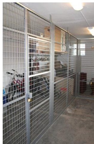
After renovation – basement storerooms
