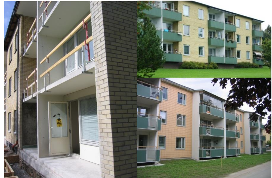
Long side façade with balconies before (left and above) and after (below) renovation.
