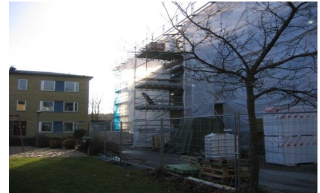
During reconstruction the building was covered by a tent.
