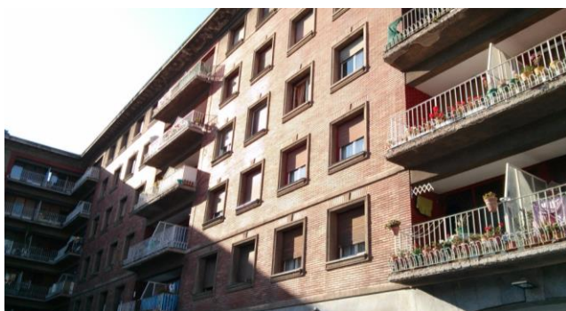
Building façade before renovation
