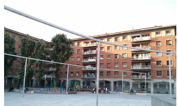
Building before renovation
