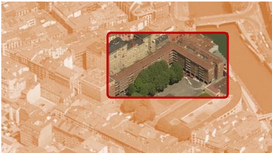
General view of the building
