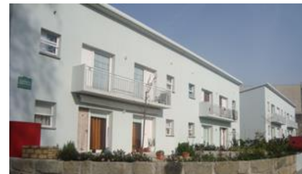
Building after the renovation process
