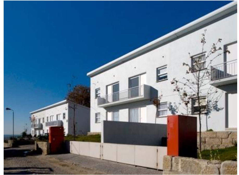
Front facade of the renovated buildings
