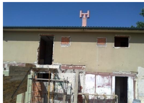
Building during the renovation process
