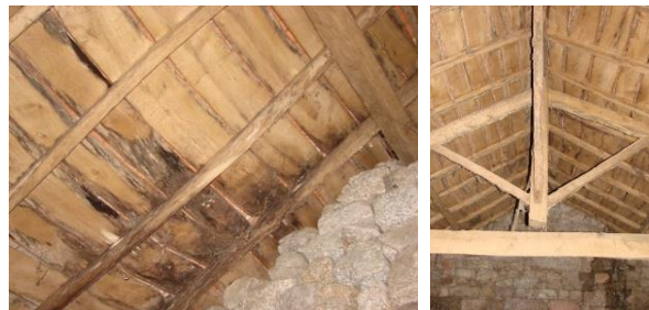
Roof condition and characteristics
