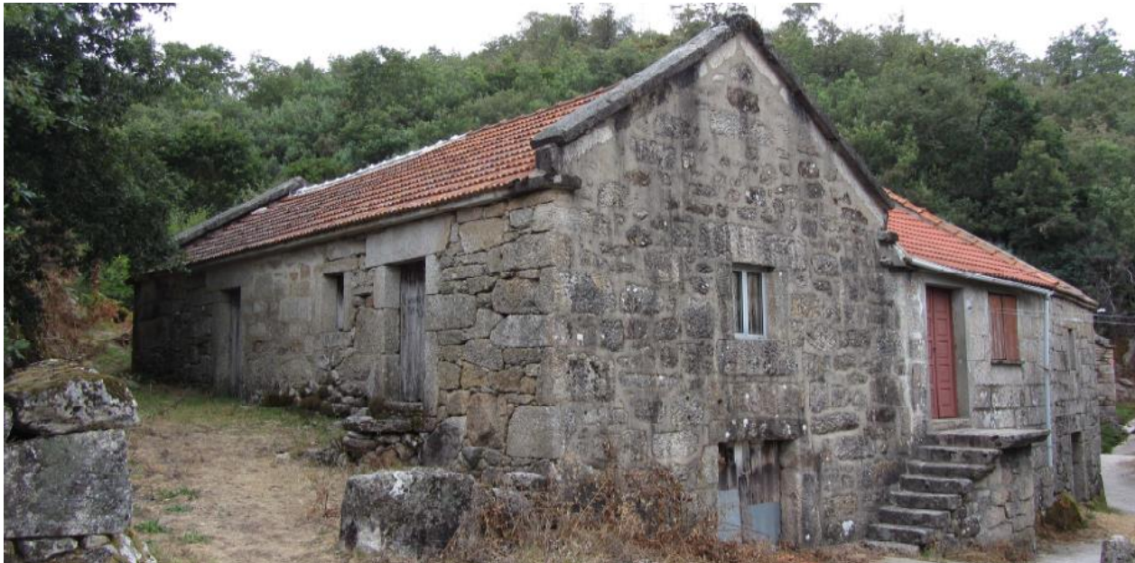
Country house before intervention (south east and southwest facades)
