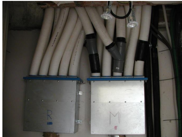
Distribution section of mechanical ventilation system.
