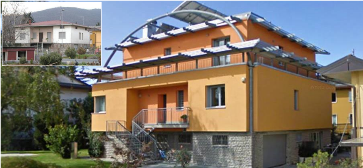
View of the building before (small picture) and after renovation (large picture ).
