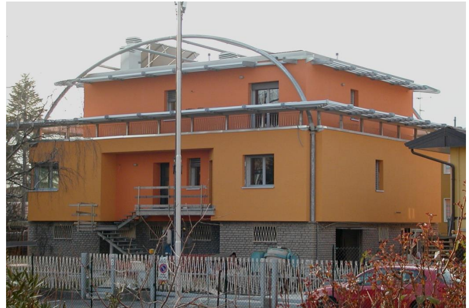
View of the building during renovation.
