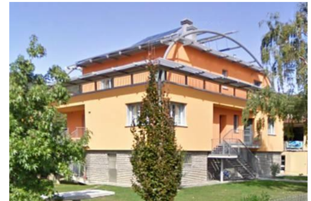
View of the building after renovation.
