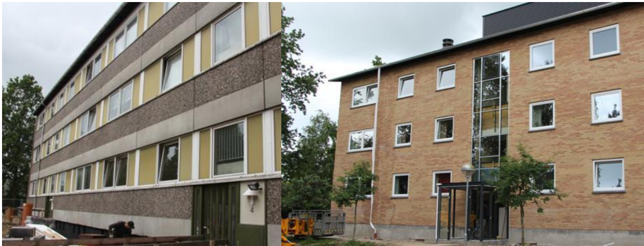
2 of the 3 blocks at Traneparken. The one on the left not yet renovated – the other after renovation.
