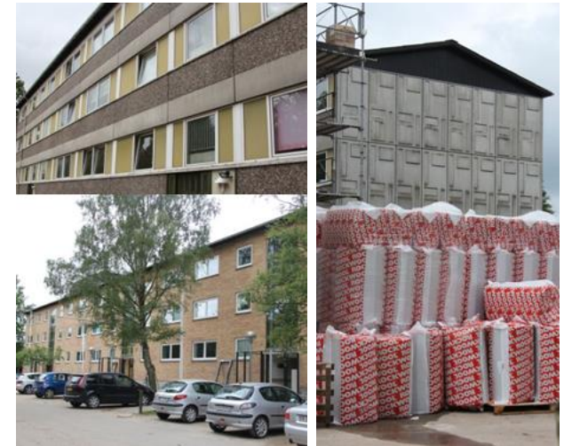
Facades – before and after
