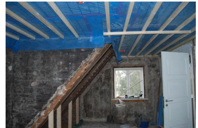
The new vapour barrier on the loft
