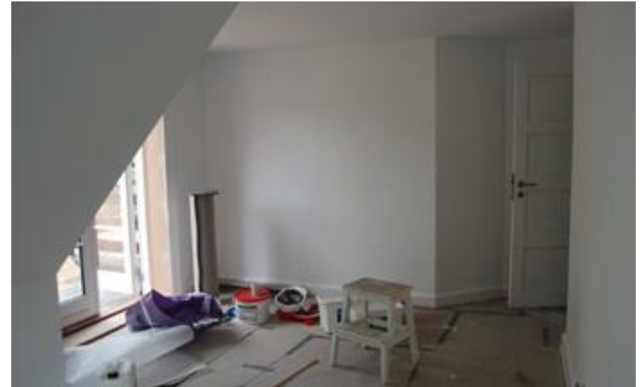
Pediment in the bedroom with new balcony door - almost ready to move in.
