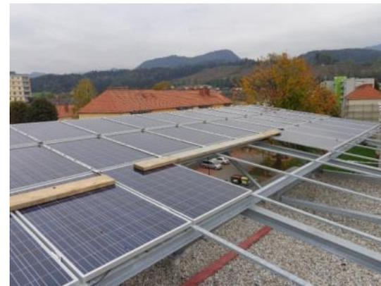
*Mounting of the photovoltaic panels on the roof (left picture), pv and solar thermal panels on the south façade (right picture)*
