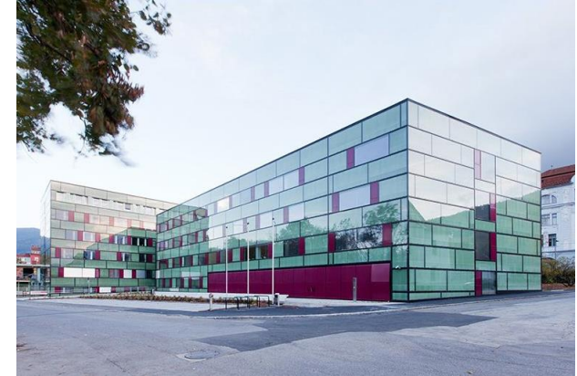
Building after the renovation (© Markus Kaiser, Graz)
